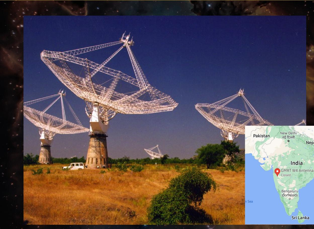
An array of 30 steerable parabolic telescopes, each of 45 m diameter Spans over 25 km, provides a total collecting area of about 30,000 sq. m at metre wavelengths, with a fairly good angular resolution (~arcsec)
